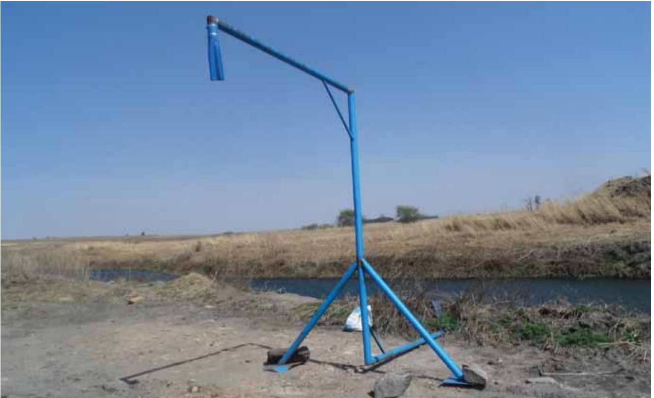
Permanent pump next to dammed Wilge River which contractors use to extract clean water for mining at Delmas Coal
