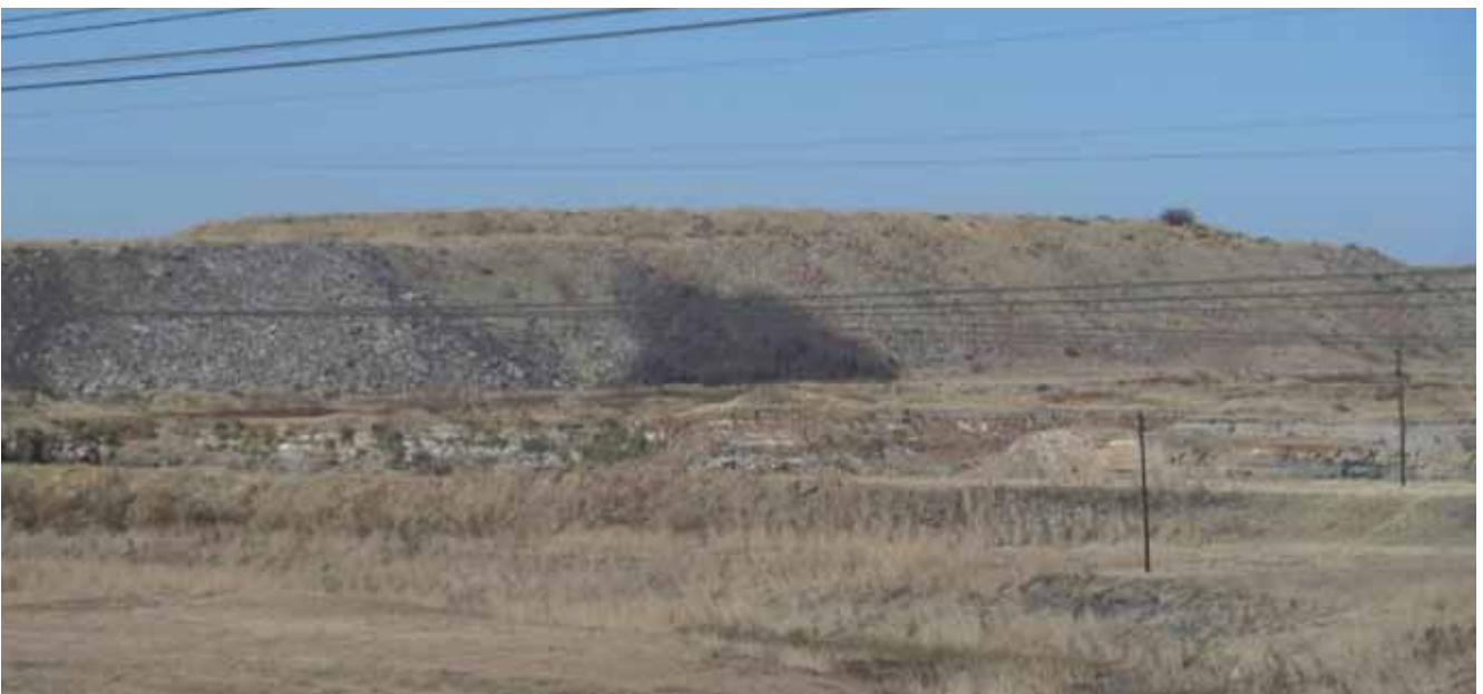
Abandoned, unrehabilitated mines left by previous owners on the property of Delmas Coal. Rain flows over the discard in a process of Acid Mine Drainage which the Wilge River carries downstream.
